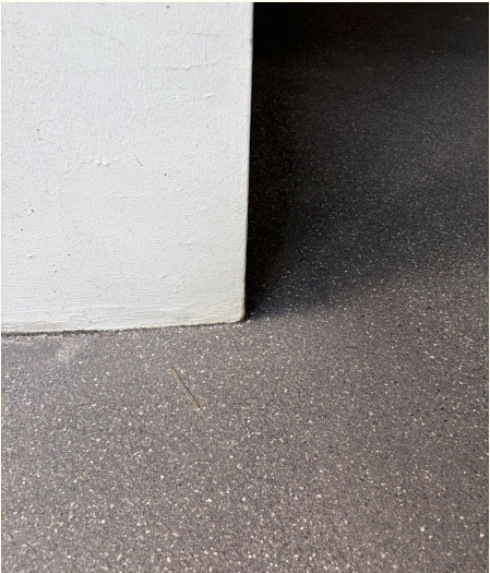
Epoxy Flake Floors at Void Decks
